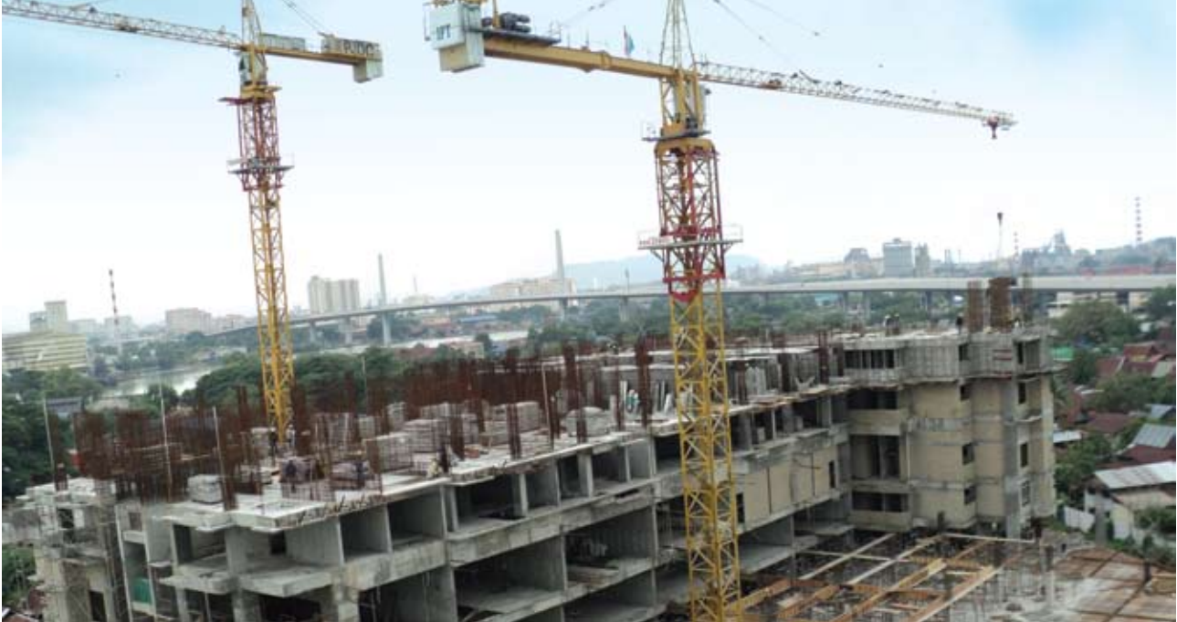
Construction in progress
